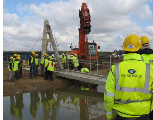
Figure 7 Brewery Wharf bridge
