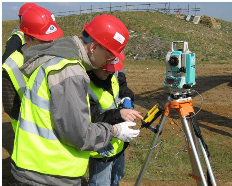
Figure 3 Setting out using LM 80
